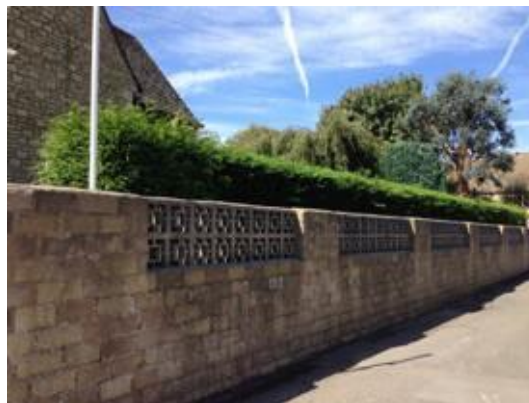
Near left, 5.12.9 Boundary, concrete block wall with trellis effect in Back Lane, replaced a dry Cotswold stone wall. The lane marks the boundary of the Conservation Area. (FNP12 No.5, 6)
